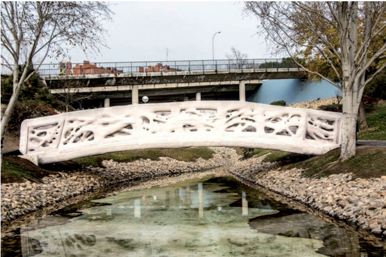
FIGURE 3.10: 3D PRINTED 12 M LONG PEDESTRIAN BRIDGE IN MADRID. Source: image provided with the permission of Acciona.
