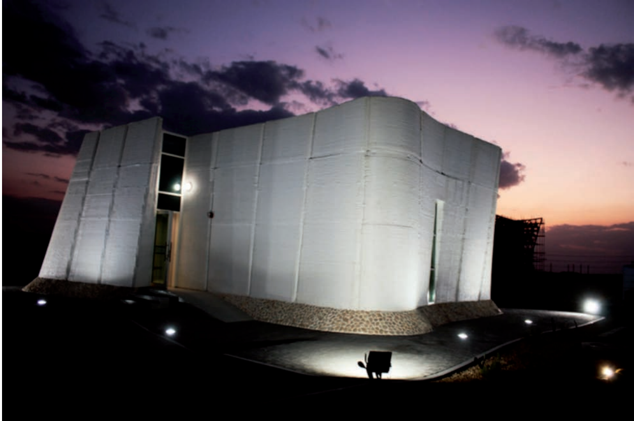
FIGURE 3.11: CYBE 3D PRINTED CONCRETE DRONE LABORATORY. Source: image provided with the permission of CyBe.
