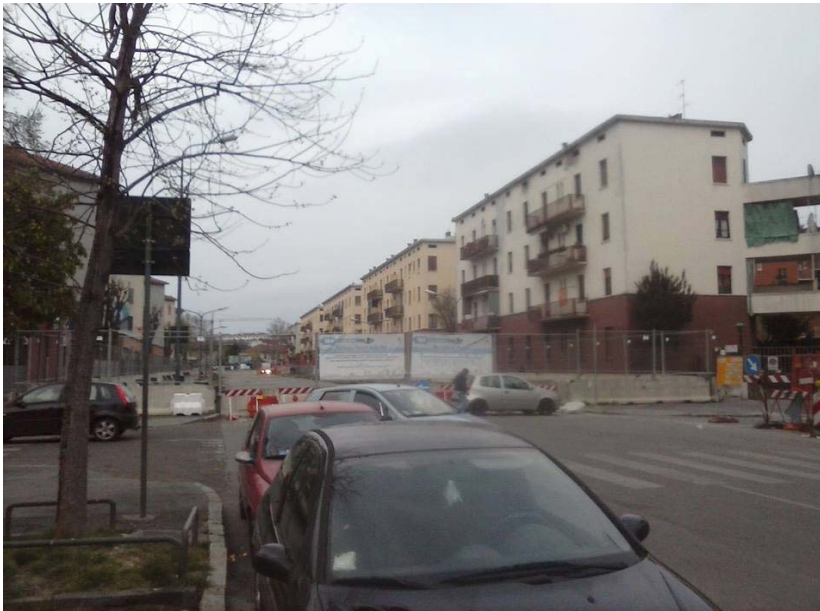
Metro line 4: work in progress
