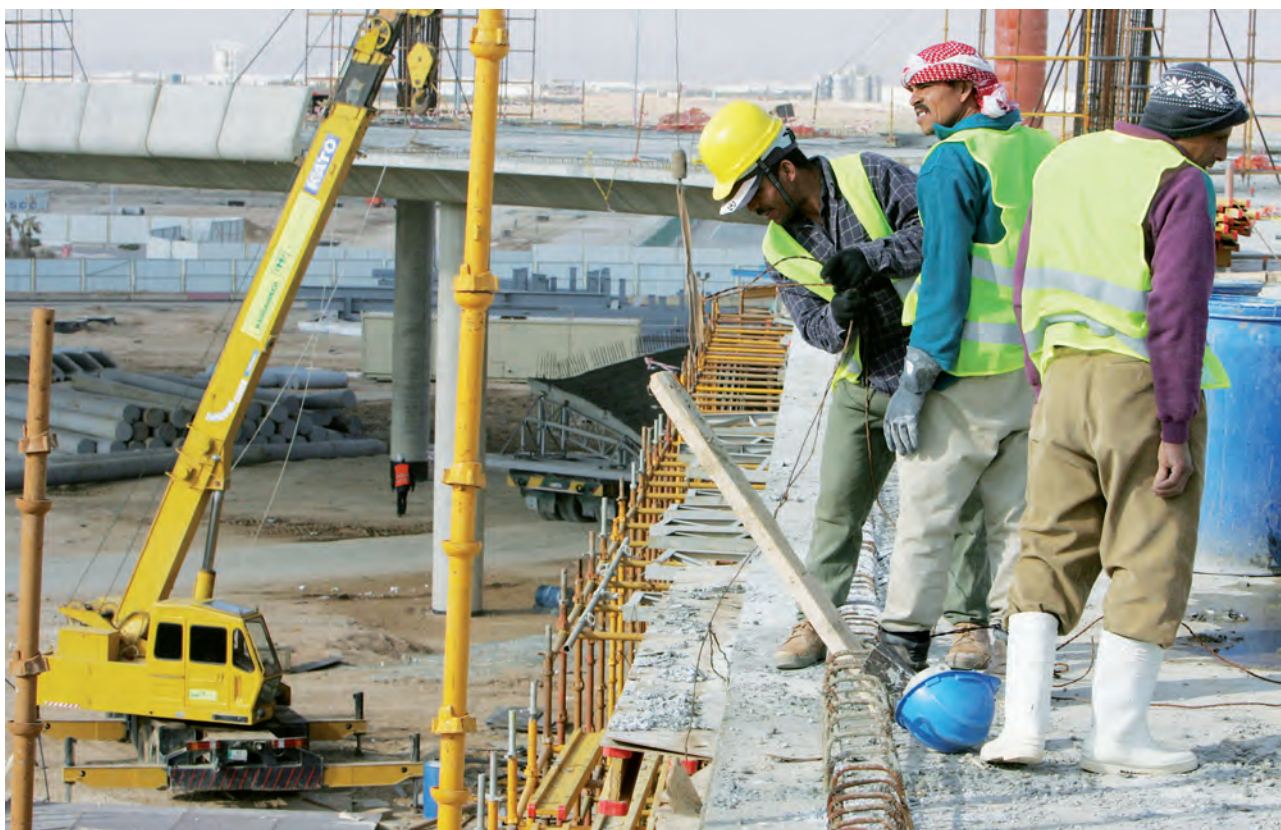
Construction workers, Gulf Region
